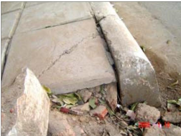
*A side view of the uncompressed loose rubble which cannot evenly support the footpath tile*
