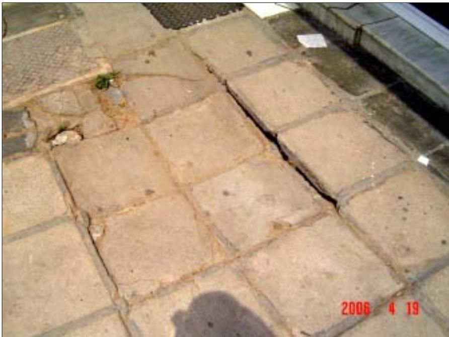
*Classic example of tiles caving in on a footpath due to uncompressed ground beneath*
