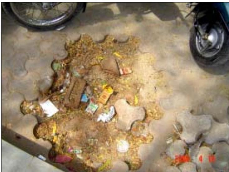
*Tiles dislodged as a result of sinking in of uncompressed ground beneath, invite garbage collection*
