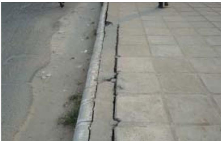
*November 2007: In time, the unsupported blocks begin to gradually fall, resulting in cracks on the top of the pavement*
