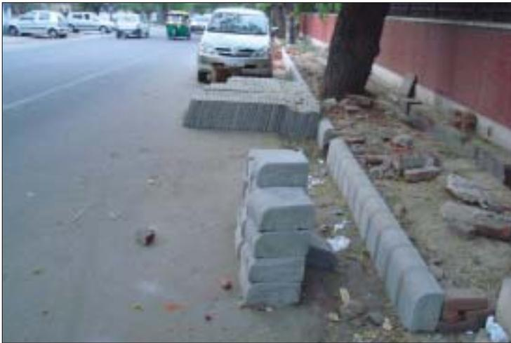
*Example of blocks placed without preparing ground or applying any adhering treatment to secure them to the ground*
