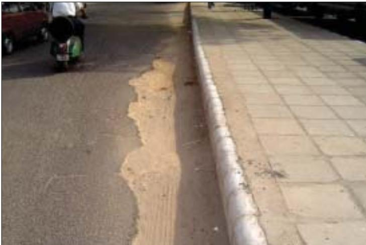
*April 2006: The tarmac on the road is not laid evenly to bleed to the edge so as to reinforce the side of the pavement*
