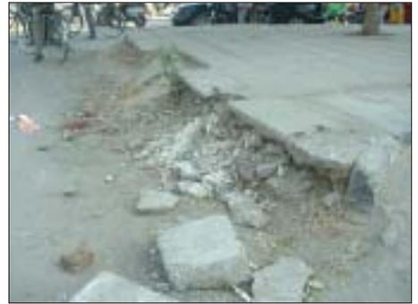
Photo document of an edge of a pavement on Aurobindo Marg that has been slowly falling apart over the last two years, littering the road with cement blocks
