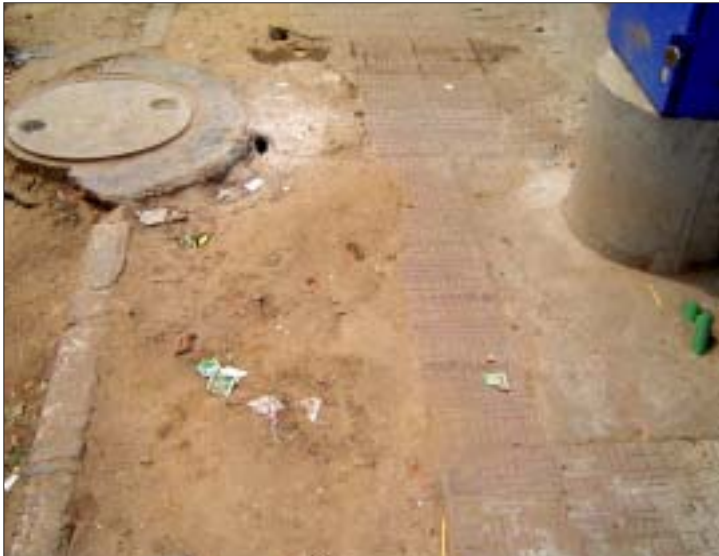
Manhole caught betwixt the pavement and the road; two mutually exclusive levels
