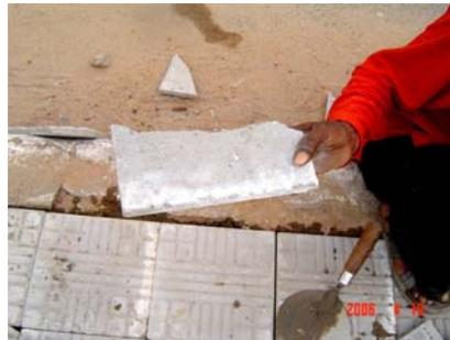
**Uneven edge of paving tile broken with inappropriate tool**
