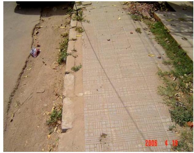
A gap left between edge of pavement and tiled area as tiles could not be cut to size.
