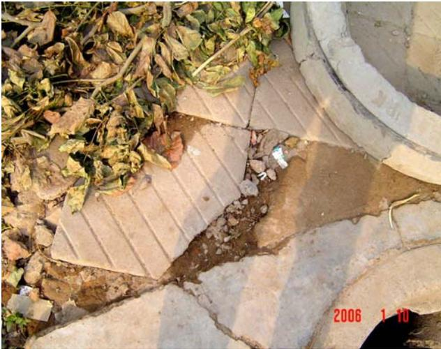
Close up of an unevenly cut tile that is not secured and hence can come off easily.
