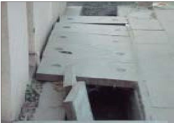
Brand new slabs fall into the drain. Note, that there is absolutely no margin to support the slabs on one end
