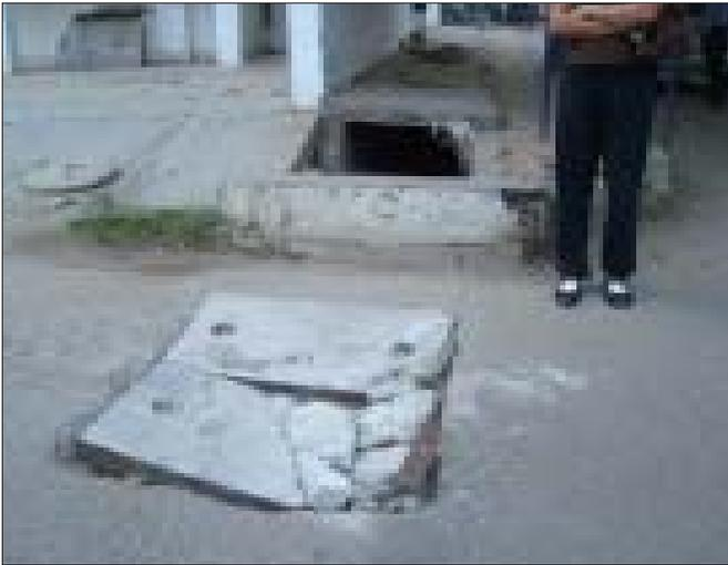
**Caved-in drain slabs with sharp metal edges, hazard for motorists and pedestrians alike**
