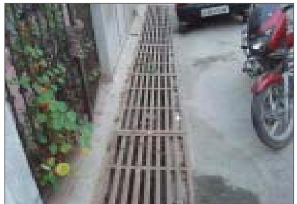
**A metal drain cover on hinges: a good workable option**
