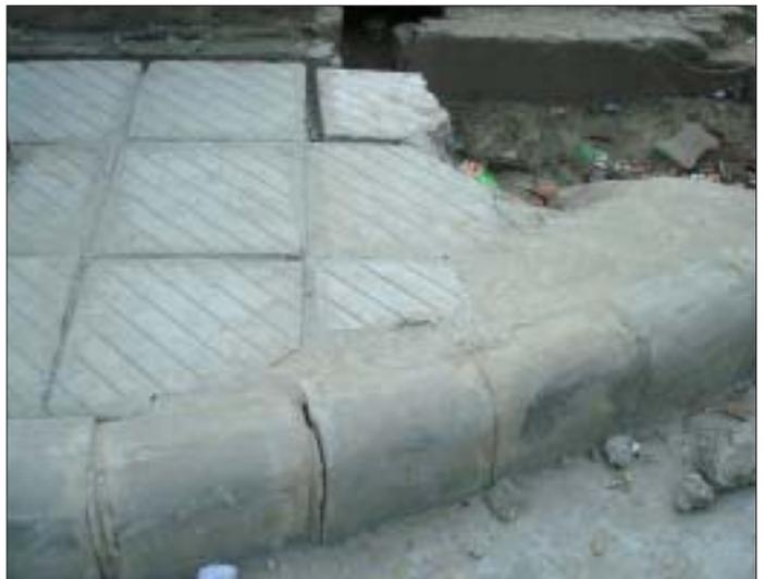
*Edge of pavement that has to negotiate the ill-defined road, plinth of the house, a rainwater drain, and the curve, 'completed' on August 27, 2008*
